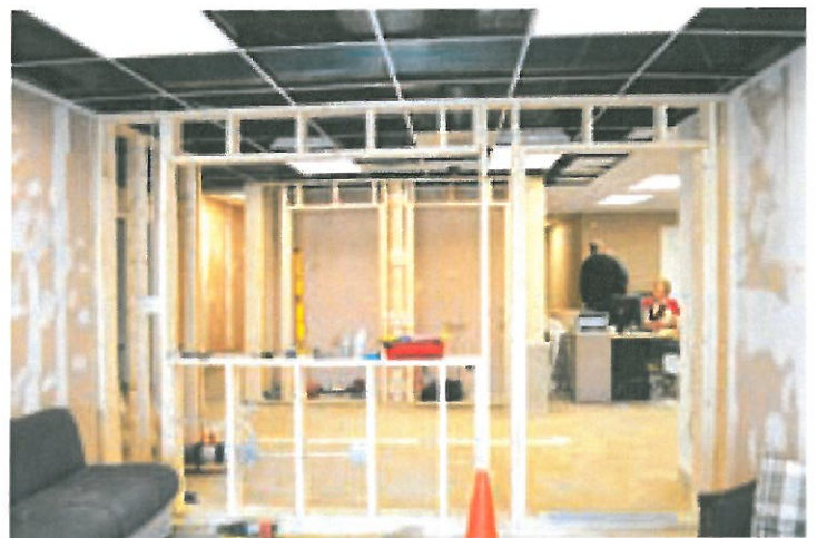
Renovations at the Township's Mental Health Resource Center
